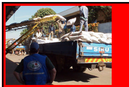
Conveyer to truck loading
