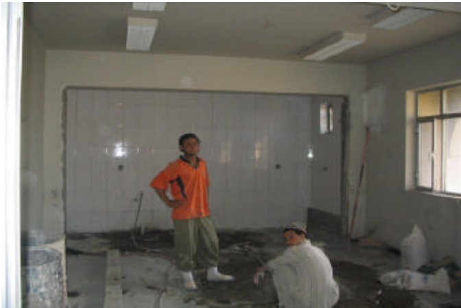
The look of the hospital during rehabilitation
