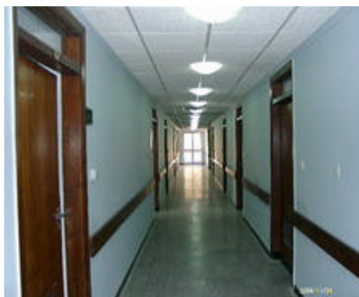
The newly-finished interior of the IRCS maternity hospital (Phase I).
