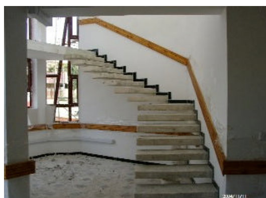
The PSP Centre in Suleymaniah, November 2004, now completed.
