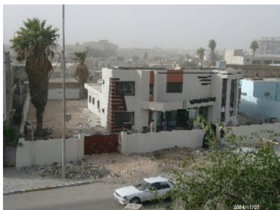
Basrah PSP Centre, November 2004, now completed.
