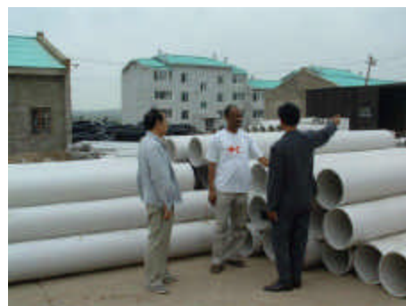
DPRK Red Cross trained local technicians to install water and waste water pipes and fittings.
