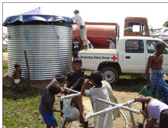
The German Red Cross ERU produces 110,000 litres of drinking water daily. (Photo Konrad Kerpa GRC)
