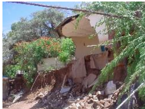
Floods in Hargeisa destroyed hundreds of houses and basic infrastructure.
