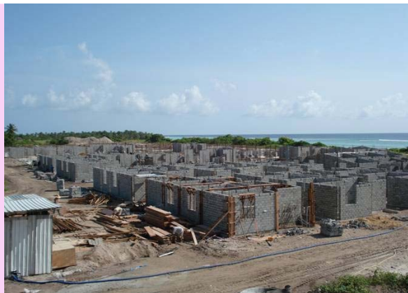
Construction of 400 to 600 houses underway on the island of Dhuvaaafaru
