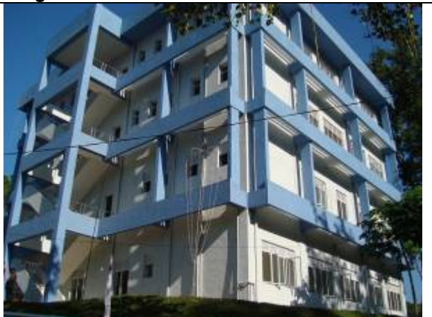
As part of the International Federation's construction and rehabilitation of health facilities in Sri Lanka, Kamburupitiya base hospital, in the district of Matara was built with the generous funding and technical support of the French Red Cross, together with the SLRCS, and implemented by the IFRC. The Red Cross set about in enhancing Kamburupitiya hospital's capacity to act as a secondary referral hospital in the area while at the same time, improving the quality of patient care provided.
