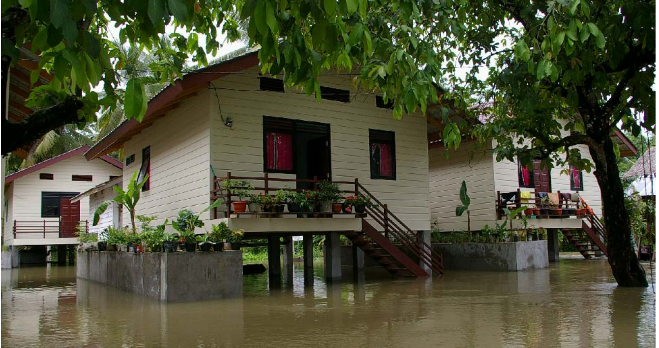
Elevated houses along with sanitation systems designed for flood prone areas in Indonesia. Nigel Ede/ British Red Cross
