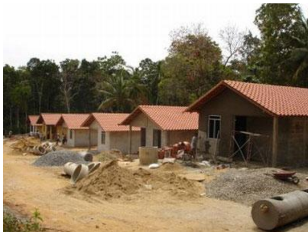
Red Cross Red Crescent construction site in Matara where 18 houses have been built and are now ready for occupation.
