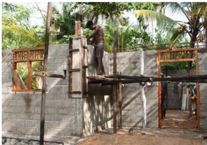
Construction of one of 52 homes being built by the Belgian Red Cross (Luxemburg), in Beruwala, Sri Lanka
