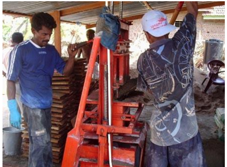
Beneficiaries running the block making project in Akkaraipattu Sri Lanka are producing 1,000 blocks each day
