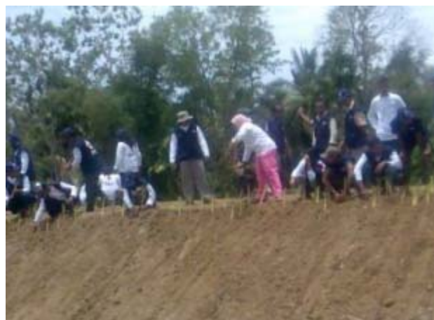
PMI and village volunteers plant protective grass on a newly built dyke in Teunom as part of the Danish Red Cross ICBRR programme in Aceh. Danish Red Cross/
