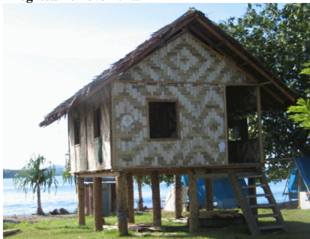
A completed medium-term shelter. These shelters are relatively sturdy, spacious and have proper ventilation.
