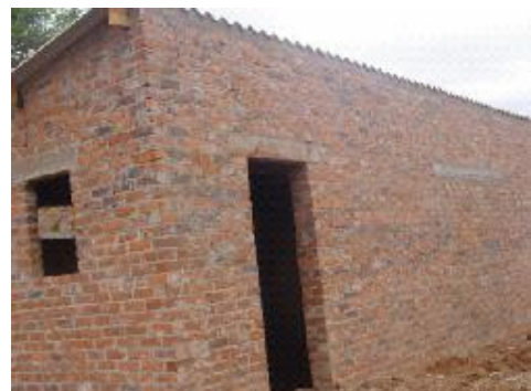
One of the houses under construction in Hatcliff, Harare
