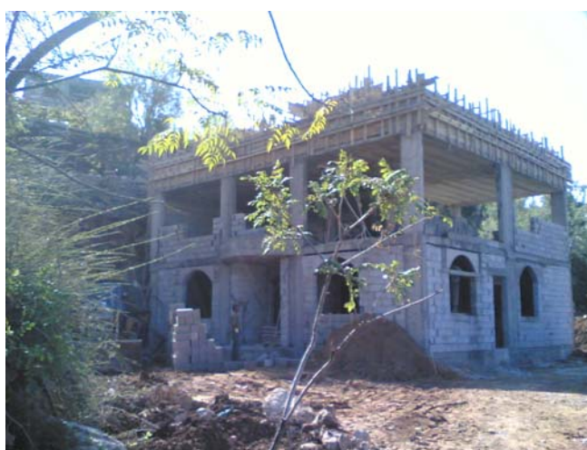
Construction of the emergency medical service station in Kabr Chmoun
