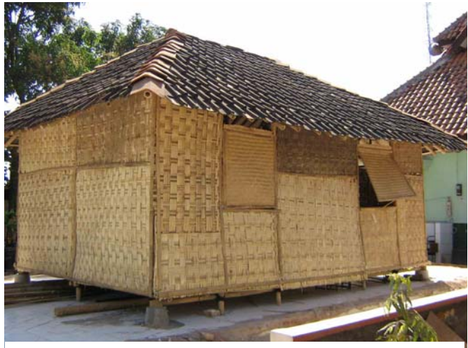
A completed model temporary house constructed utilizing locally available bamboo and local craftsmen. The house can be constructed in five days at the cost of 150-200 USD and lasts for 3 to 5 years.
