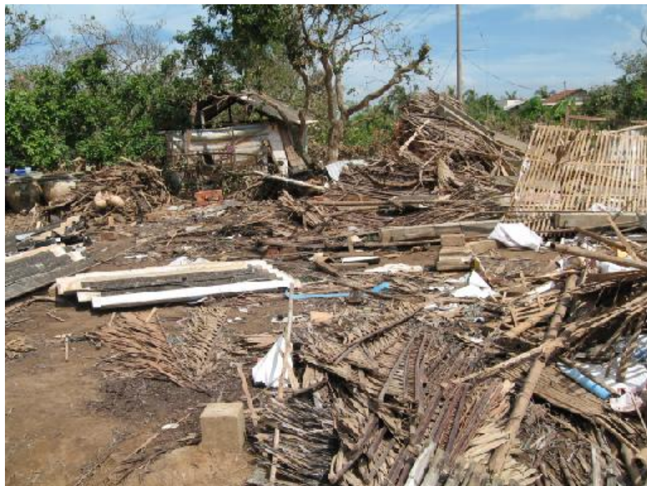
The typhoon devastated homes with poor people being particularly affected.
