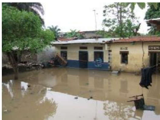
Flooded house in Kinshasa
