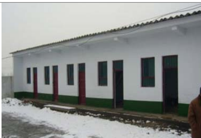
A collective house block of five in Shuanglou Village in Henan province is nearly ready for the families to move in.
