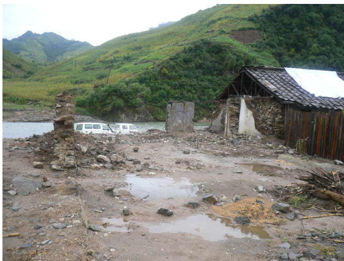
An assessment team of DPRK RC and Federation staff visit Maengsan county to assess the damage caused by the flood. Federation/Peter Kurlandsky
