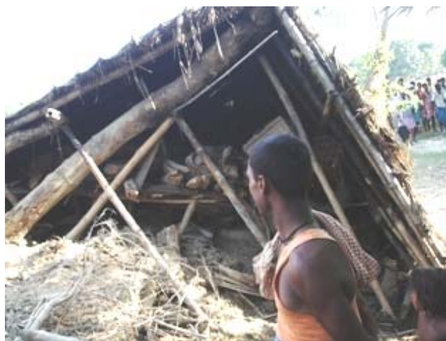
A youth observing his collapsed house in Dhanusa district, eastern Nepal.
