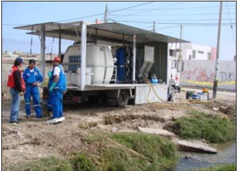
PRC's water treatment plant in Pisco. Source: International Federation.
