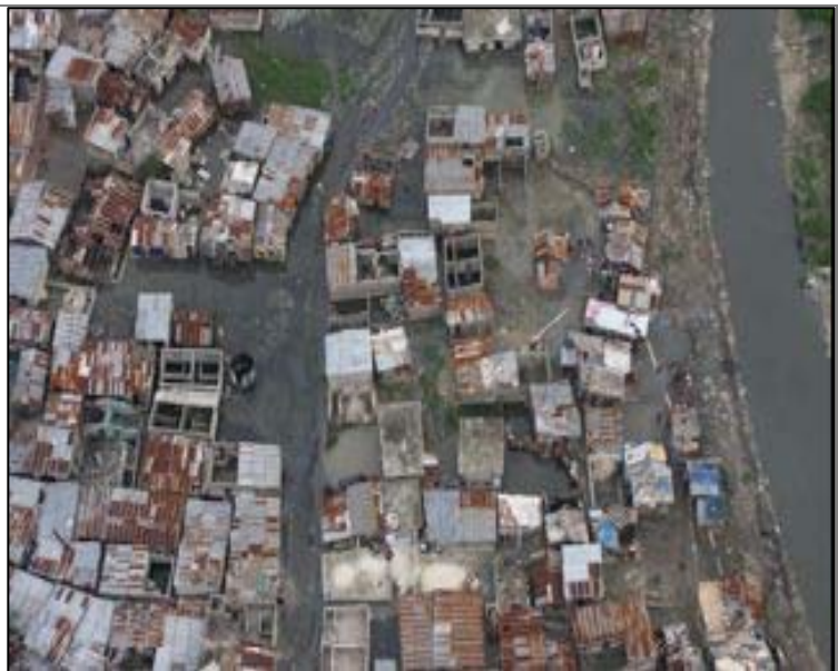
The extensive damages to roof tops in Haiti became clear during an air assessment. Source: International Federation and American and Spanish Red Cross.
