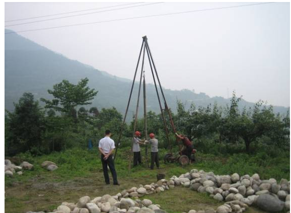
Geotechnical survey at new water treatment plant site. Photo: RCSC
