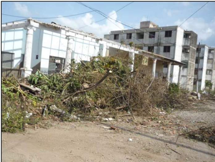
Debris caused by the storm in Municipality of Los Palacios. Source: International Federation
