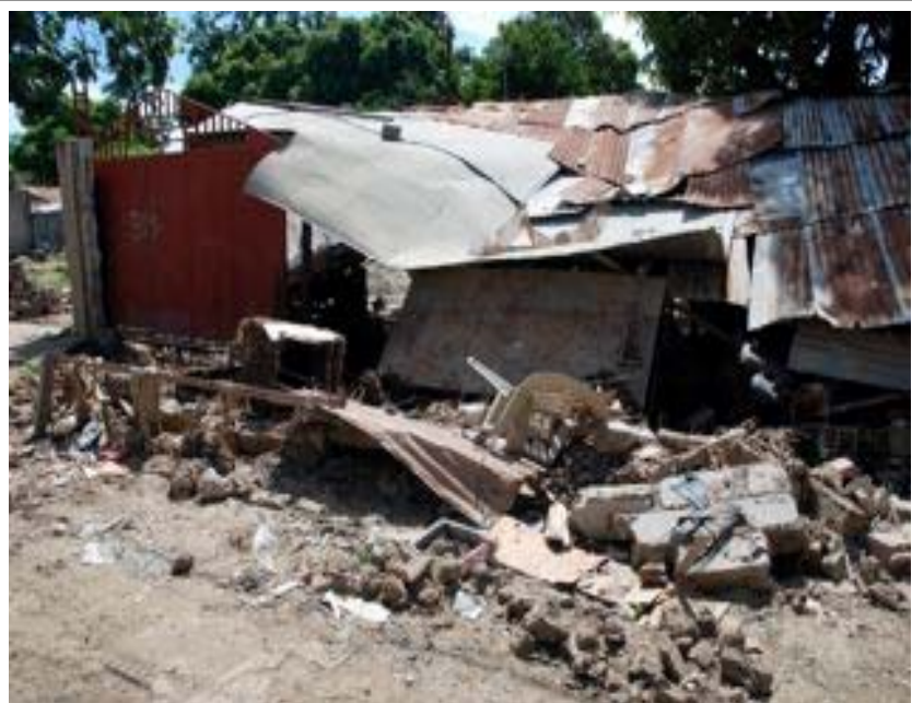
One of the many destroyed houses demonstrates the urgent need for construction materials. Source: International Federation
