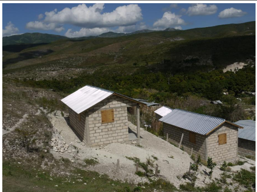
400 new storm-resistant houses were built under the shelter programme. Families whose houses were completely destroyed were able to re-build their homes under the ‘build back better’ community-based approach. Source: International Federation/I. Marin
