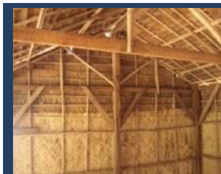
A timber framed house featuring wall corner-bracing.
