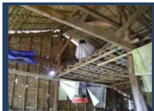
Some houses include storage space in the roof which can be useful during flooding.
