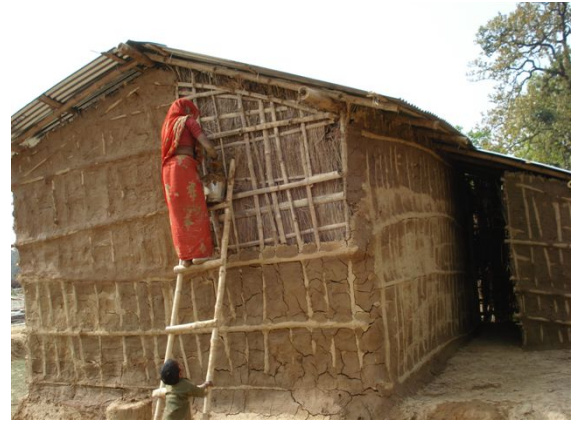
Beneficiaries were involved in constructing their own houses, with support from the NRCS and International Federation.
