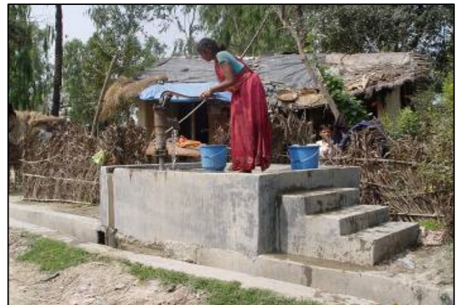
Community water sources were repaired/installed in selected vulnerable communities.
