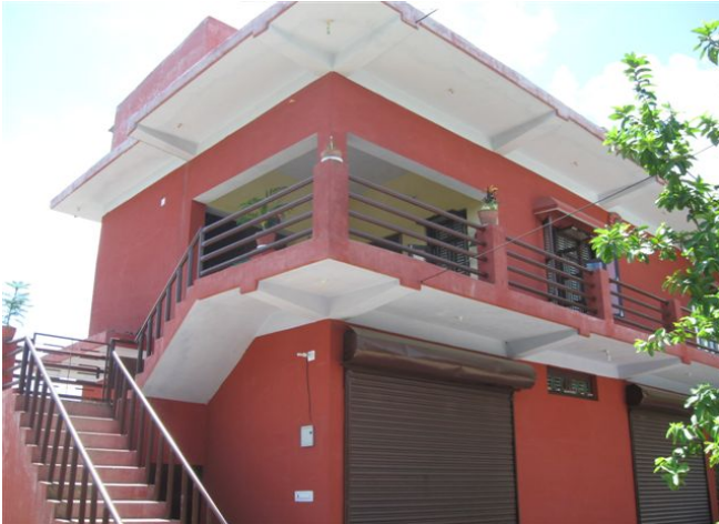
NRCS has repaired and constructed different ten warehouses
