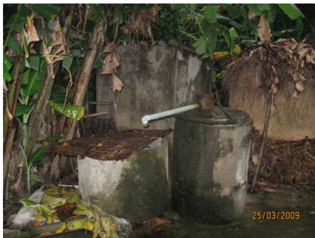
In Thanh Nguyen commune, Ha Nam province, households that experience floods regularly have taken to using water tanks such as these. Tanks are tightly lidded with plastic to keep floodwaters out. Once floodwaters have receded, lids are removed and the household has access to water at least for several days. (Photo: VNRC, Ha Nam chapter)
