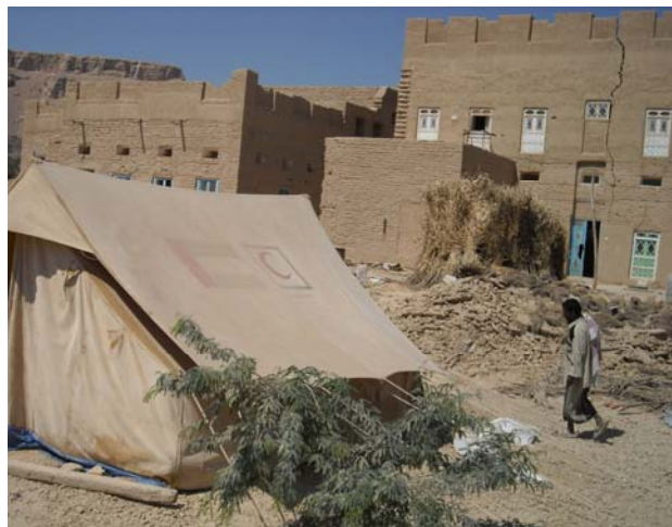
The floods of October cracked or destroyed houses in south eastern and south western Yemen
