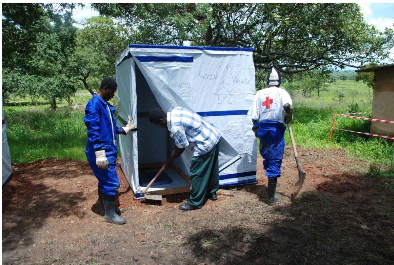
One of the temporary latrines constructed at the CTCs
