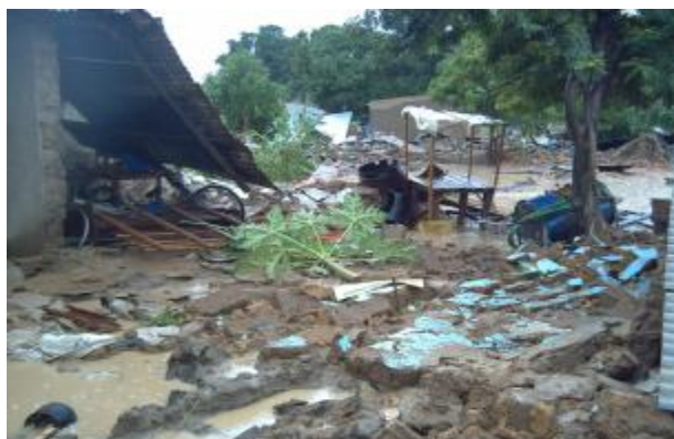
Remainder of collapsed houses in flooded areas.
