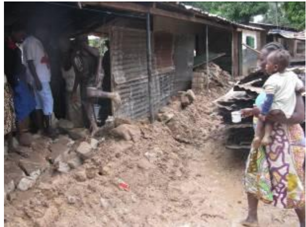
Many houses like this one have been destroyed by the floods. Belly Diallo/International Federation
