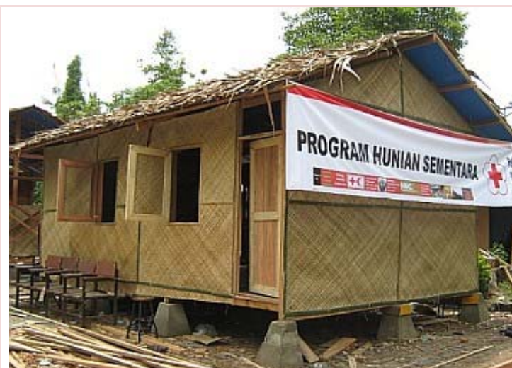
The shelter design is being finalized, with 18 volunteers receiving financial and construction training. Bill Marsden/International Federation
