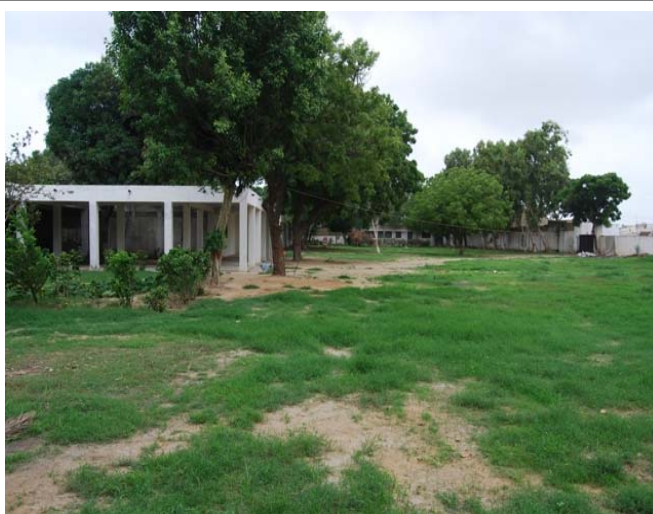
Karachi warehouse construction site. Photo: International Federation.
