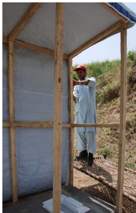
PRCS water and sanitation team constructing a latrine in Haripur.
