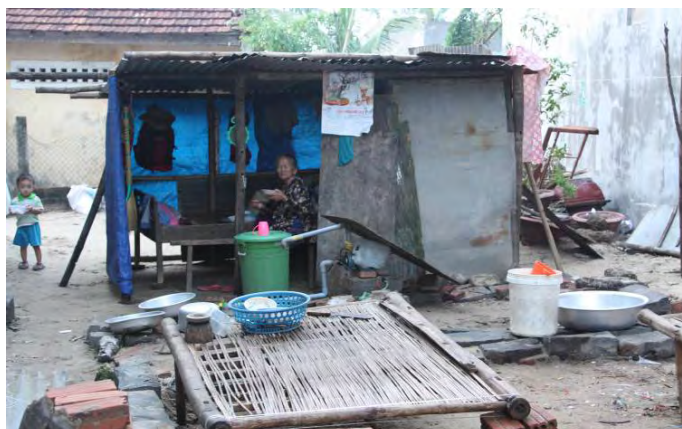
Le Thi Hong in Tan My village of Nghia An commune, Tu Nghia district of Quang Ngai province, her house was completely collapsed. IFRC
