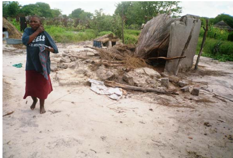
One of the damaged houses in Kweneng district
