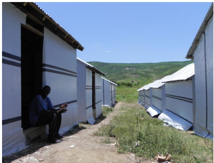
These transitional shelters were built by the IFRC in the northern town of Saint Marc on land provided by a local NGO. Land ownership is a major issue which has slowed the process of building shelters.
