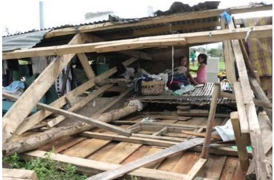
Children seek shade under the remains of what used to be home. Their home was among the 25,000 destroyed in Isabela. Photo: Hajime Matsunaga/IFRC
