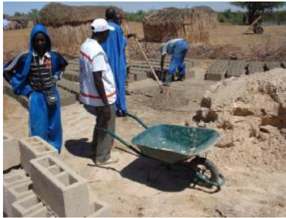
Beneficiaries using kits to rehabilitate their damaged houses
