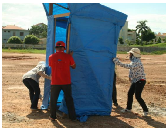
Building an emergency toilet was part of practical exercises carried out during the water and sanitation training in Quang Binh and Da Nang provinces last August. (Photo: VNRC/IFRC)
