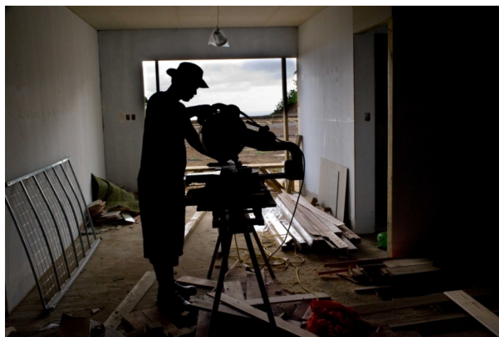
Housing construction continues
