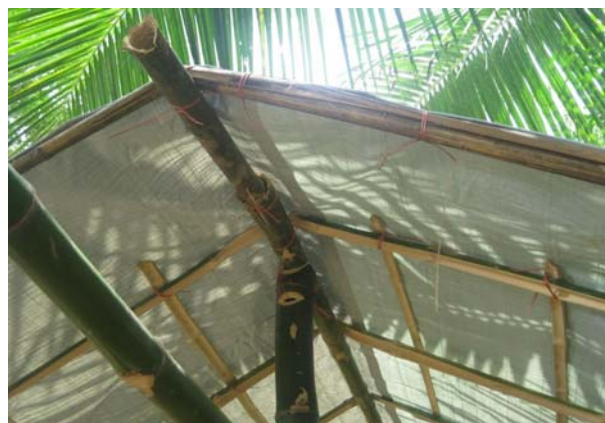
Use of locally available bamboo and rope to fix tarpaulin in Cox's Bazar. Photo: IFRC
