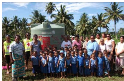
With the completion of the main water system and reallocation of a 5000L community tank, children of Saleamua preschool now have access to clean and safe water. Photo by SRCS.
