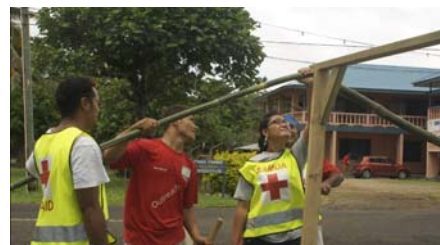
SRCS volunteers combine local materials such as bamboo with the standard shelter kit tools to construct a safe emergency shelter during five day shelter kit training. Photo by Tania Ahmed SRCS.
