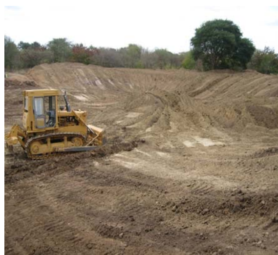
In Machakos, an arid area of Kenya, surface dams are being constructed to better utilize scarce rainfall for vulnerable communities. Kenya and Spanish Red Cross Societies
