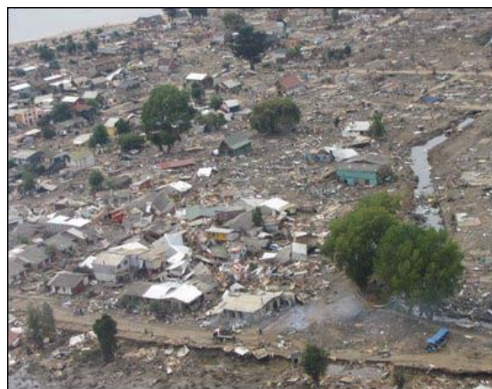
Aerial assessment after the earthquake on Talca and Concepcion in Chile (March 2010). IFRC
