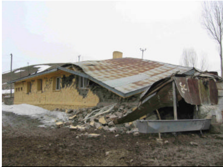
Devastation: In Karabiyik several buildings were badly damaged.
