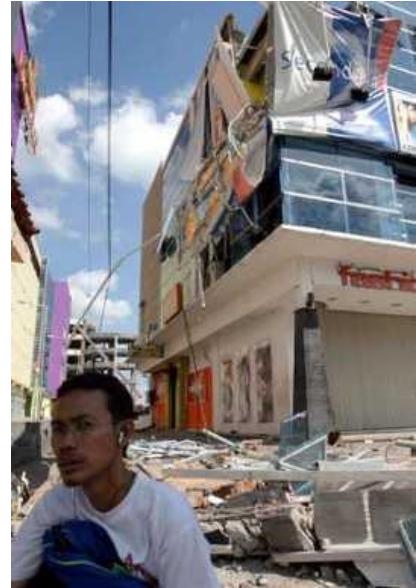
Indonesian man stands in front of damaged shops in Yogyakarta
